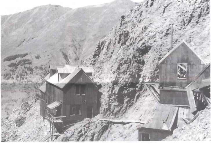
gallon buckets and then walk through the building and dump them out the windows." Crews had to rope off while working on the roof or risk a couple thousand foot roll into Cunningham Gulch. Contractor Loren Lew had to put the finishing touches on the lower roof while being belayed. Other work included the Colorado Division of Minerals and Geology installing a gate at the portal of Seven level.
