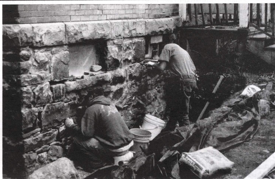
Foundation work on the jail continues on the outside, stabilizing the old structure to a far better degree than it has ever been and preventing further moisture incursion.
