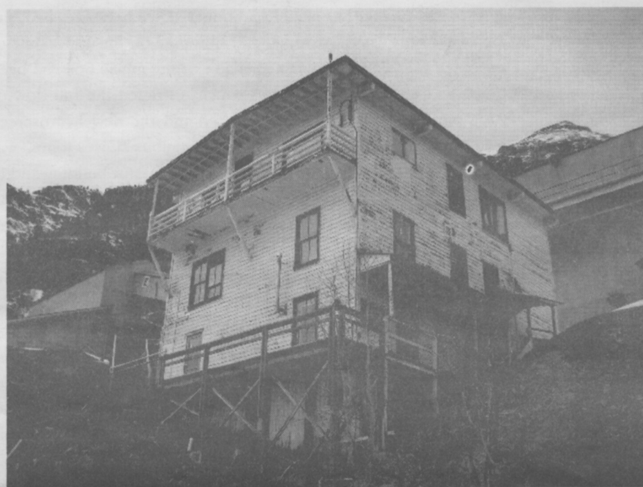
Suffering from severe problems after years of neglect and ill-conceived repairs, the assay office building will be the subject of a two step restoration, starting with the exterior.
