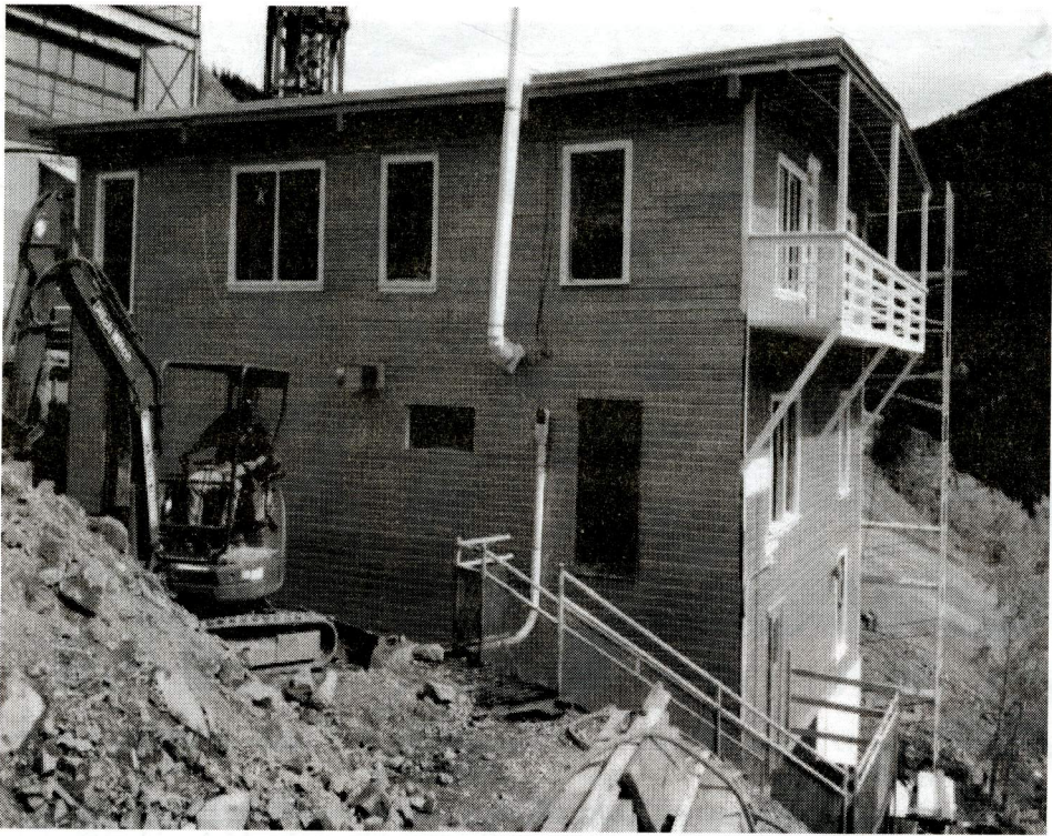
The assay office building at the Shenandoah Mill site will serve the Society in a number of ways once the restoration is completed. Here Donny Curnow is operating the backhoe, improving the drainage around the building.
