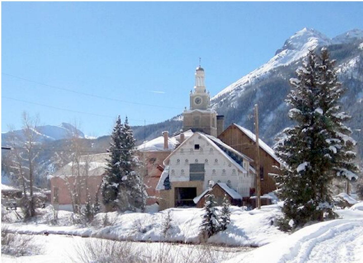
The extent of the new addition to the Mining Heritage Museum is obvious in this mid-winter view from Memorial (formerly Lions) Park. To the immediate left is the Jail Museum and to the left of that, the Allen Nossaman Archive.
