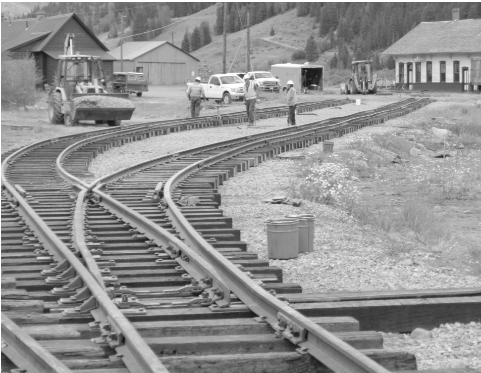
Shown here are switches and track laid by Savage Services. Installation of ballast should be completed this summer
