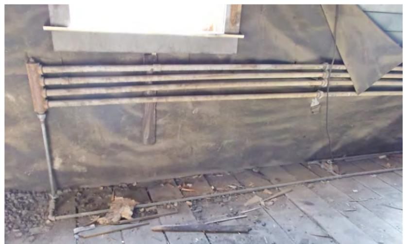
*Working with buildings that have been around more than a century uncovers a lot of mysteries like this piping network along the east and south walls in the engine house back room. It appears to be heating pipes along east wall and spray pipes on floor along both walls. True purpose is unknown and it is too modern for the period of significance – they were removed.*
