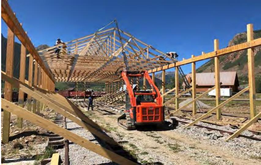
*Crew from National Barn Company of Colorado Springs works on erection of the 40.5 by 224 foot Railcar Shed which will not only protect completed restorations but provide space for restoration work on additional cars in the future. Elevated platforms will provide both visitors and workers easier access to the cars.*
