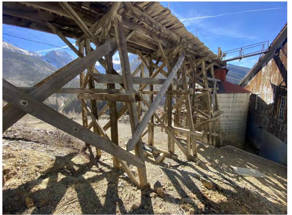
The massive trestle and coal tank will be receiving attention and restoration in the latest phase of the Mayflower Mill restoration efforts over the next year.
