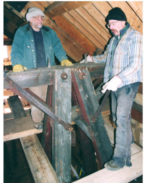
Jerry and Scott Fetchenhier installing a mine frame in the Mining Museum.
