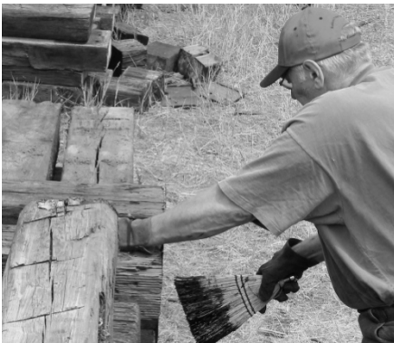
2009: Jerry paints the end of a narrow gauge tie, cut down from standard gauge size, with asphalt foundation coating.
