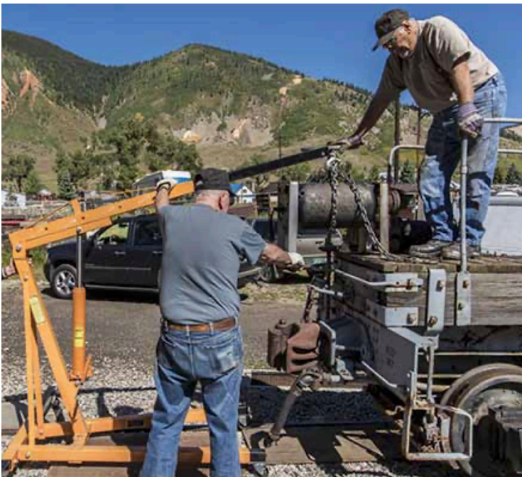
2015: Jerry and Duane Danielson maneuver the brake reservoir and mounting brackets off the flanger deck so decking can be replaced.
