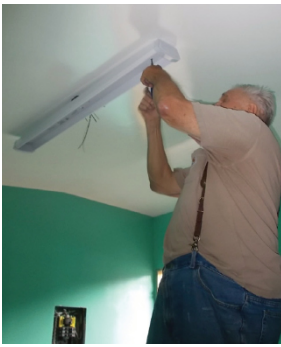
2021: Jerry installs a fluorescent light fixture in the oil shed.
